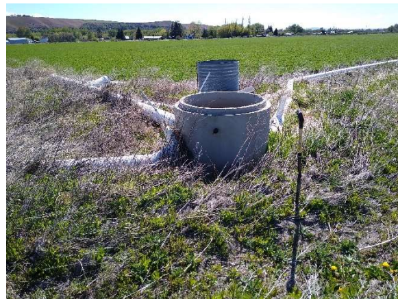
Photo 4 Irrigation weir and pipes. View toward E.
