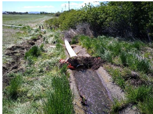
Photo 8 Gated concrete irrigation ditch to gated pipe. View toward S.
