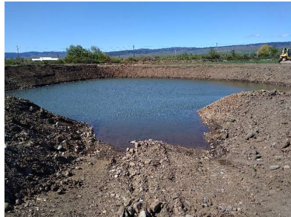
Photo 2 Excavated pond. Groundwater at ~7 ft. View toward SW.
